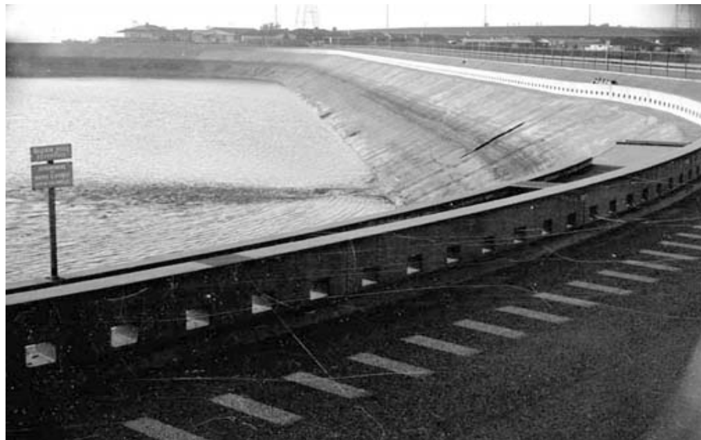
Baldwin Hills Dam - Dark spot in upper right hand quadrant shows the beginning of the break in the dam.
