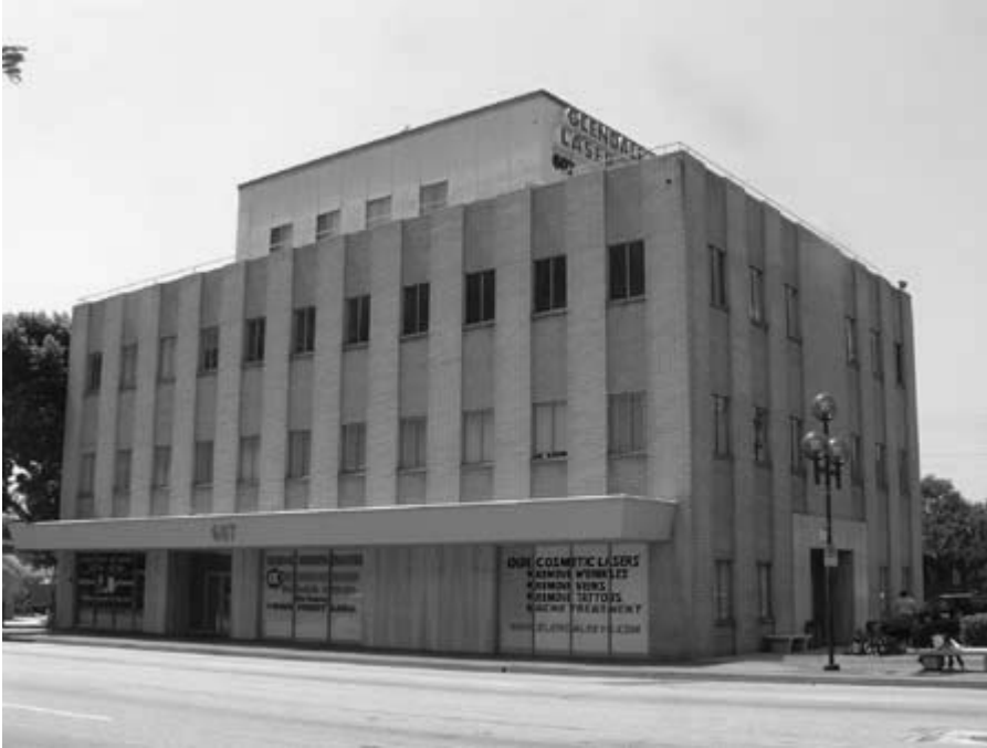
607 N. Central Avenue, East and North Elevations
