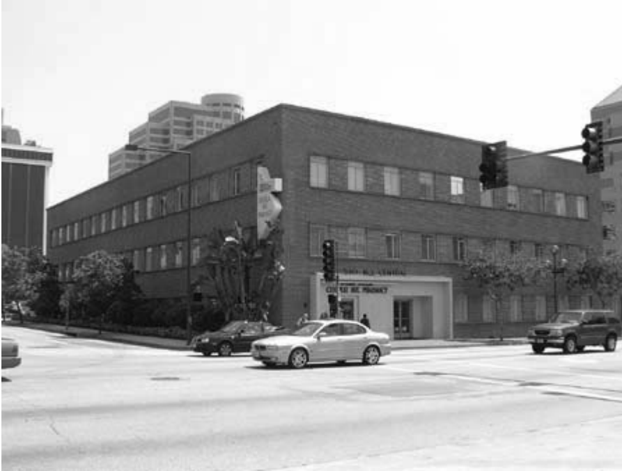
540 N. Central Avenue, North and West Elevations
