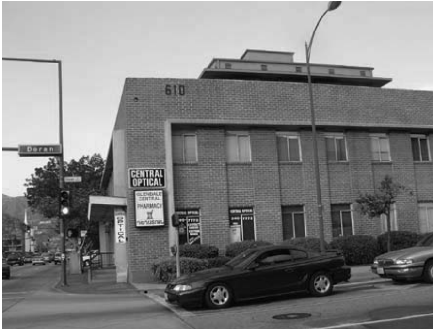
610 N. Central Avenue, South Elevation at corner of Central and Doran
