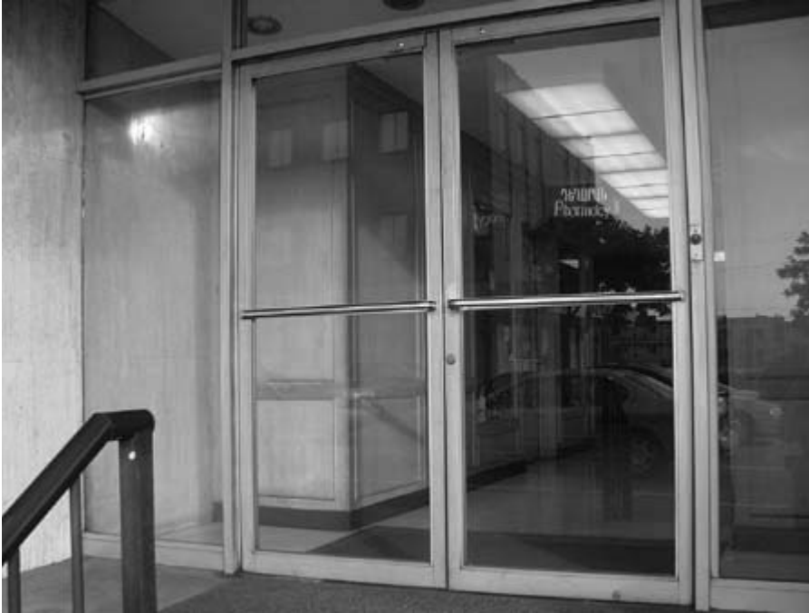
610 N. Central Avenue, Central Avenue Entry Doors
