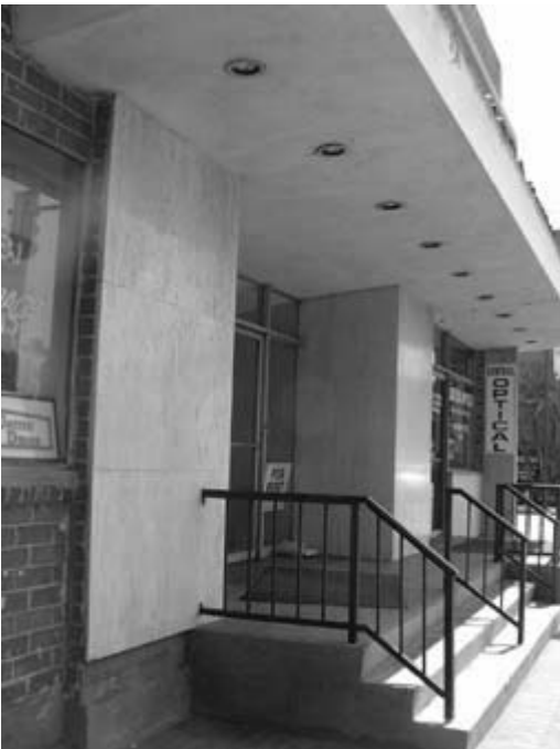
610 N. Central Avenue, Central Avenue Entry
