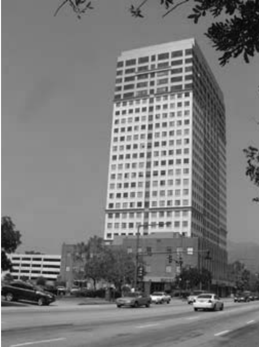
633 N. Central Avenue, South and East Elevations, with UNUM Provident Medical Center to the North
