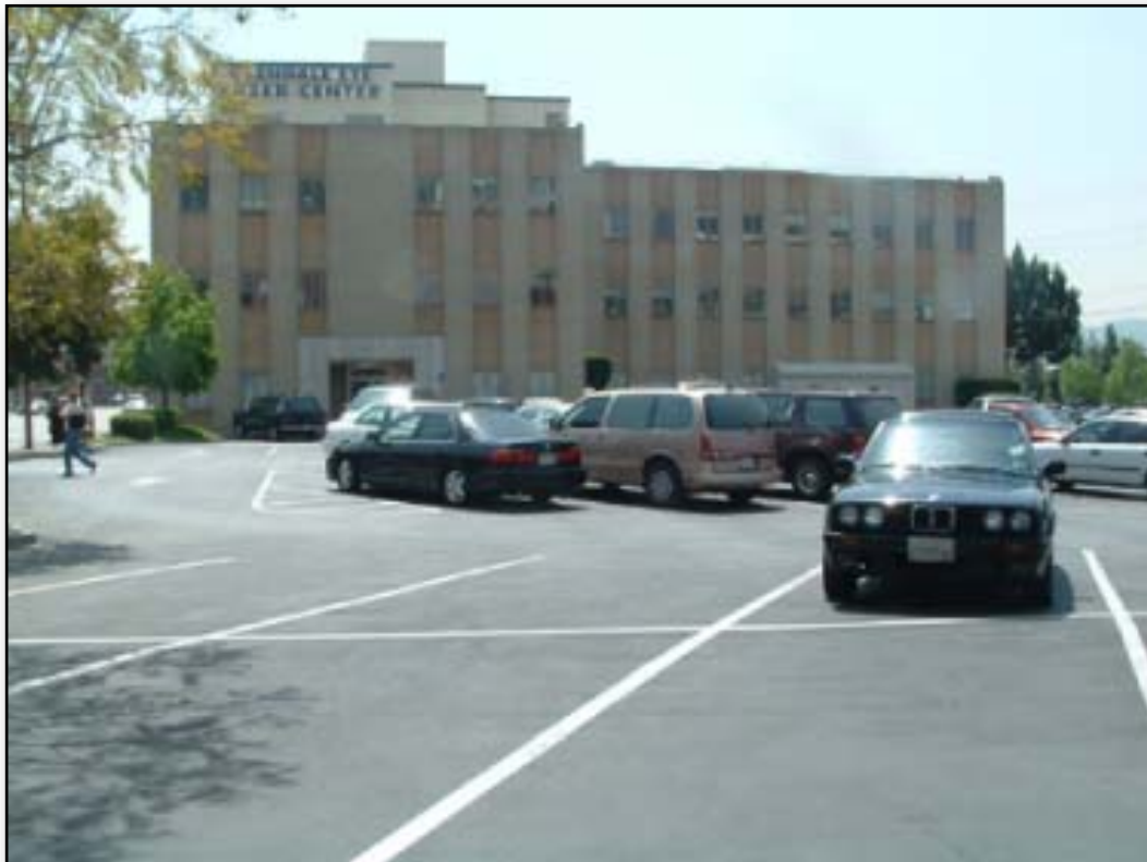
607 North Central Avenue, North Elevation (view from parking lot between 607 and 633 North Central Avenue)
