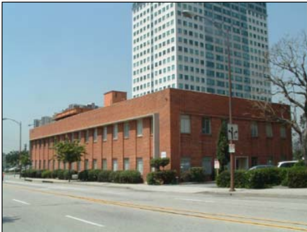
610 North Central Avenue, South and East Elevations
