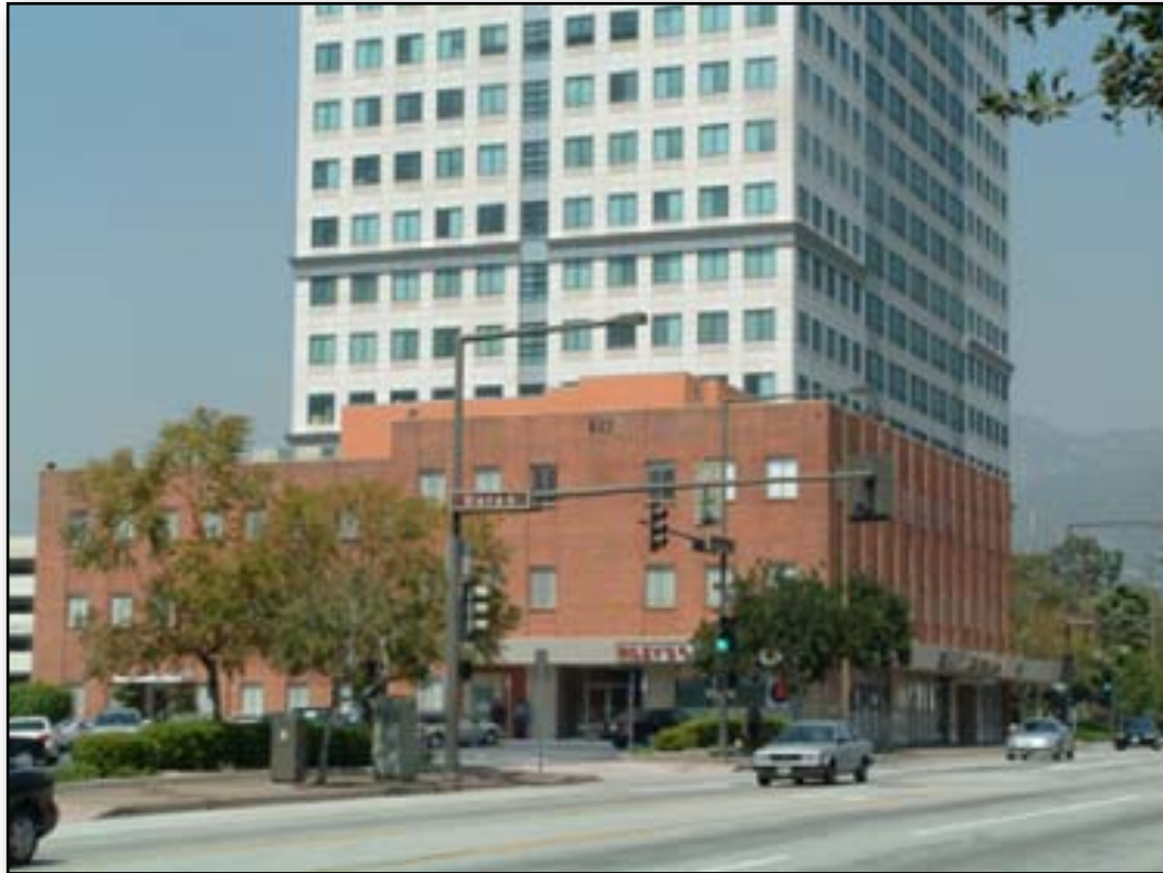
633 North Central Avenue, South and East Elevations
