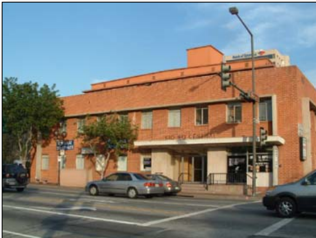
610 North Central Avenue, West Elevation
