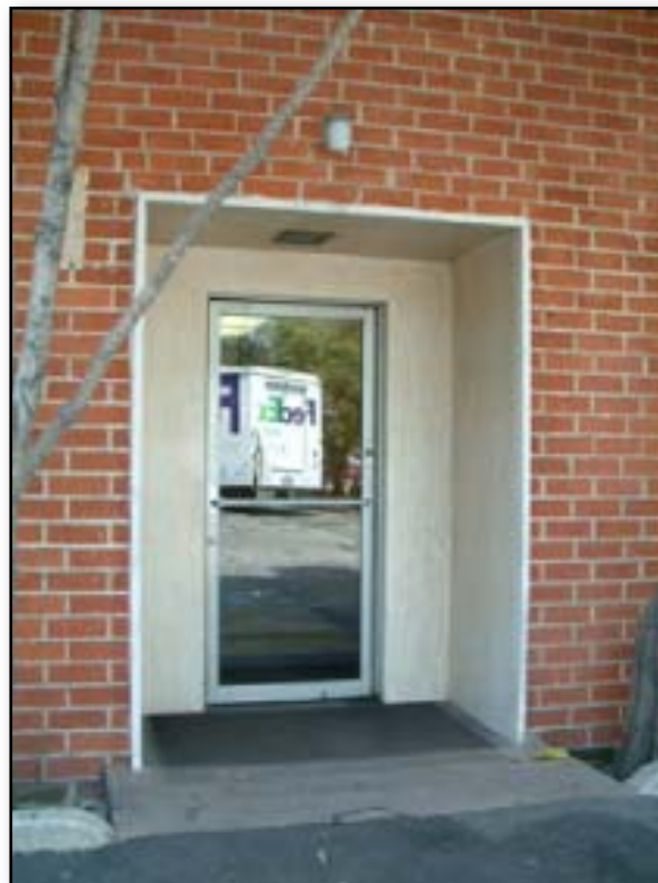
610 North Central Avenue, Rear Entrance
