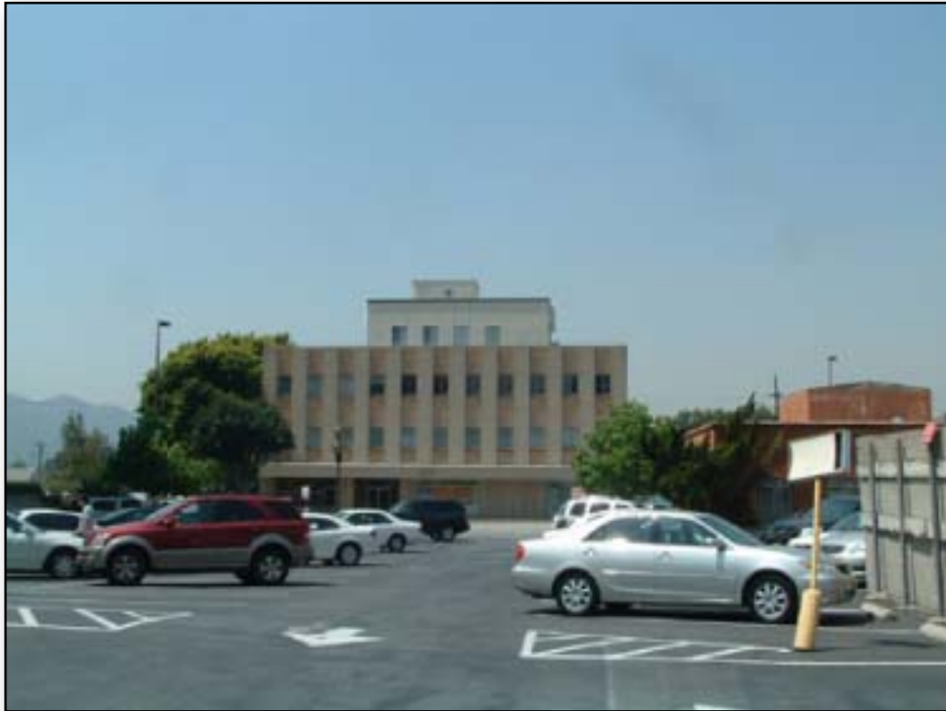
607 North Central Avenue, East Elevation (view from parking lot on east side of Central, south of 540 North Central)
